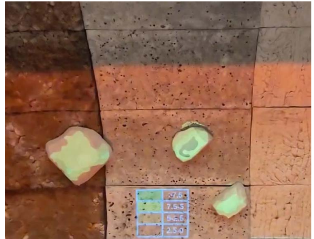
Continuous & real time display of thickness in the tunnel
